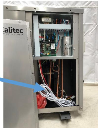
The controller needs to be connected to the outdoor unit with a 3 core cable (cable not supplied).
